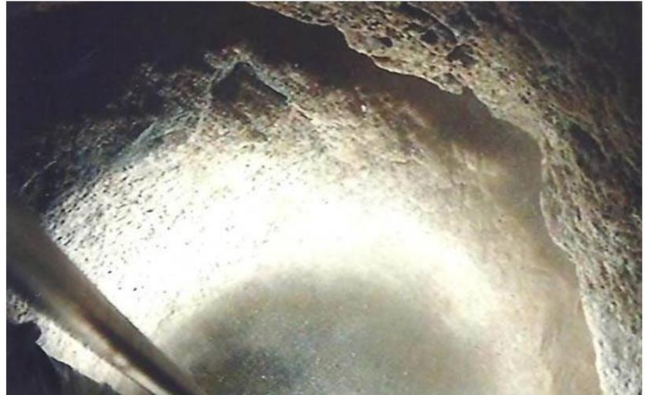
📷 Fault line: This photograph was taken by a remote-controlled camera inside the Merredin drill hole. As they drilled through solid granite at a depth of 327 metres, Globe Drill came across this fault line (seen here as a dark crack), from which water was flowing in vast quantities.
