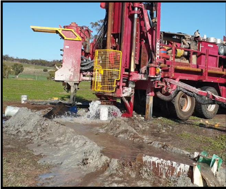
Fractured rock drilling 74m – June 2020 at York
